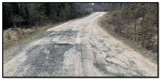
**Figure 6** – View of the road surface, especially poor section of northern portion of Whitehead Road.
